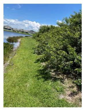
**Location 20:** Invasive vegetation growing onto pond berm. Remove approximately 5'x250' of vegetation to prevent turf deterioration/erosion.
