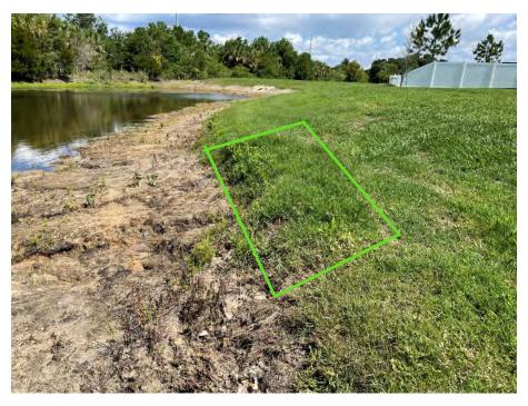
**Location 2:** 5'x5' section of pond bank is eroding underneath the sod. Restore pond bank according to attached pond bank repair detail.
