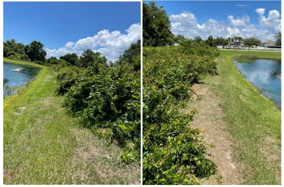
**Location 19:** Invasive vegetation growing onto pond berm. Remove approximately 5'x250' of vegetation to prevent turf deterioration/erosion.
