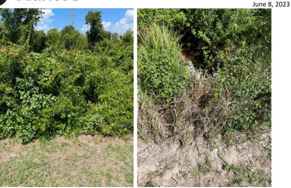
**Location 7:** Clear 6' access path and remove sediment/vegetation within 6' radius around end treatment to provide positive discharge of stormwater.
