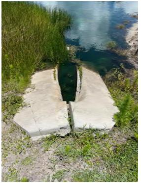
**Location 13:** Remove and replace mitered end section top. Add bahia sod around structure, with 57 stone and compacted fill beneath concrete to ensure level placement and prevent undermining/erosion.
