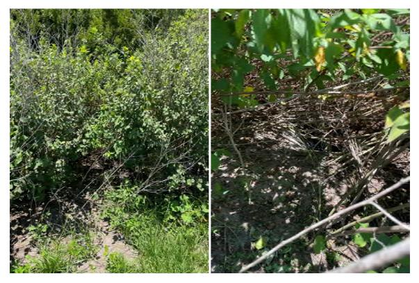
**Location 8:** Clear 6' access path and remove sediment/vegetation within 6' radius around end treatment to provide positive discharge of stormwater.
